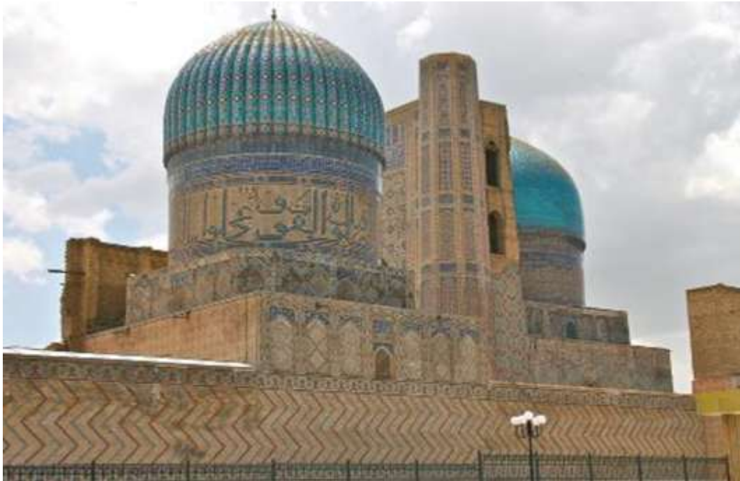
Fig 3: Exterior View of Bibi Khanum Mosque (Url-1)
