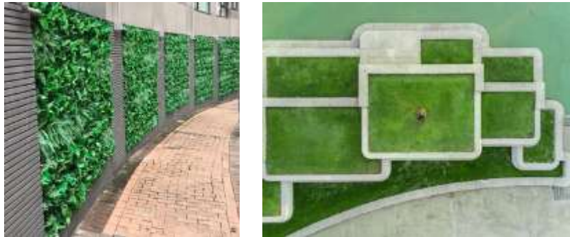
Fig 2. A greenwashed façade wall (a) and a greenwashed roof (b) [7].
