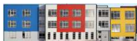
Fig. 11. North elevation of the Architecture Coloured Building (Source: Department of Architecture)
