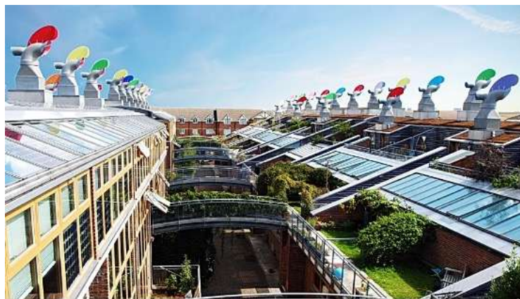
Fig. 3. Roof gardens of BedZED Ecovillage, Wallington, UK, [9]
