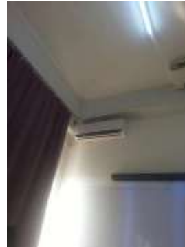
Fig. 13. A typical portrayal of blinds used internally due to lack of exterior shading devices to protect from glare and overheating. (taken by author)
