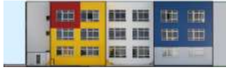
Fig. 10. East elevation of the Architecture Coloured Building (Source: Department of Architecture)
