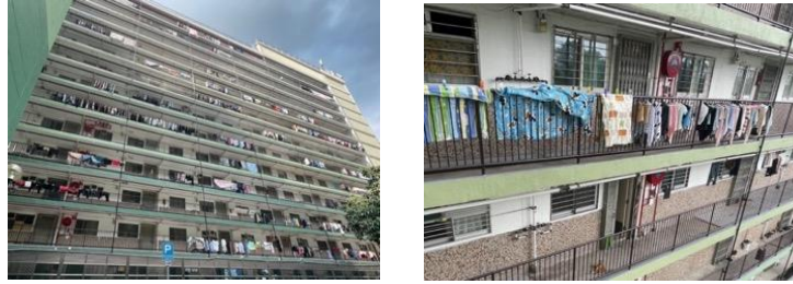
Fig. 3. Overview of the public housing complex in Hong Kong (left) and the residential shared corridor of Hong Kong (right).
