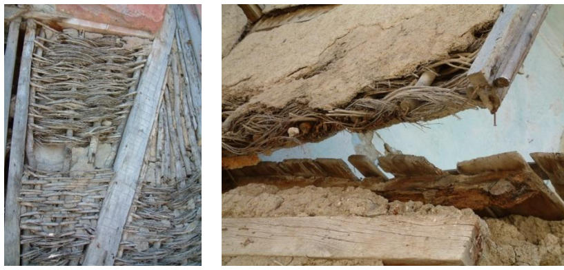
Fig.2. The branch-knitting Wall system of vernacular architecture from Ceyhan (town of Adana city) are largely seen at the districts of East-Mediterranean Region of Cukurova [Bas,D].
