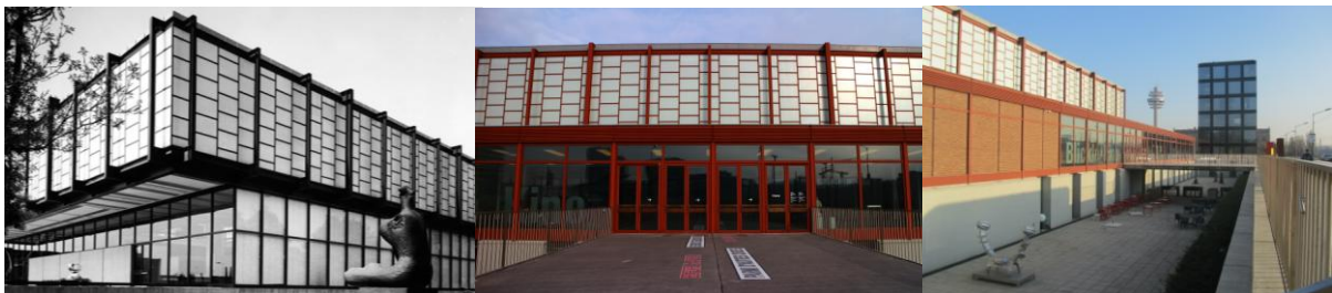
Fig. 2. (a) 20er-Haus (Photo URL [22]); (b-c) 21er-Haus (Photos by Heinz J. Selen)
