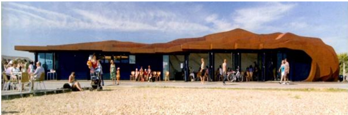
of 36 mild steel strips evoke the contours of tide-washed sand and have oil-based coating for a rust-like patina [6].
