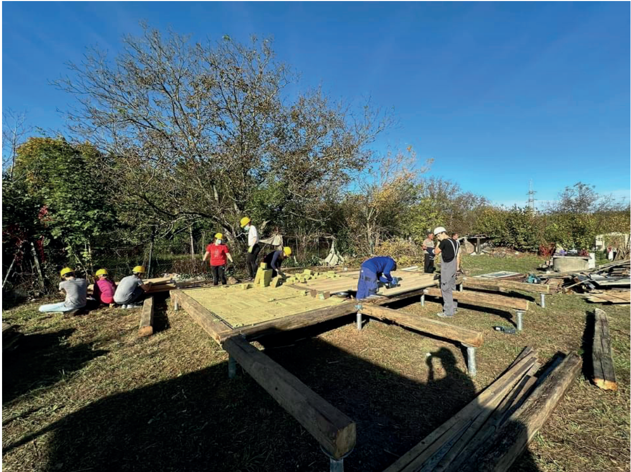
Fig. 3. The framework of the new building was made from old roof timber, lifted from the ground and attached to soil screws. The space between the beams were filled with leftover thermal insulation.
