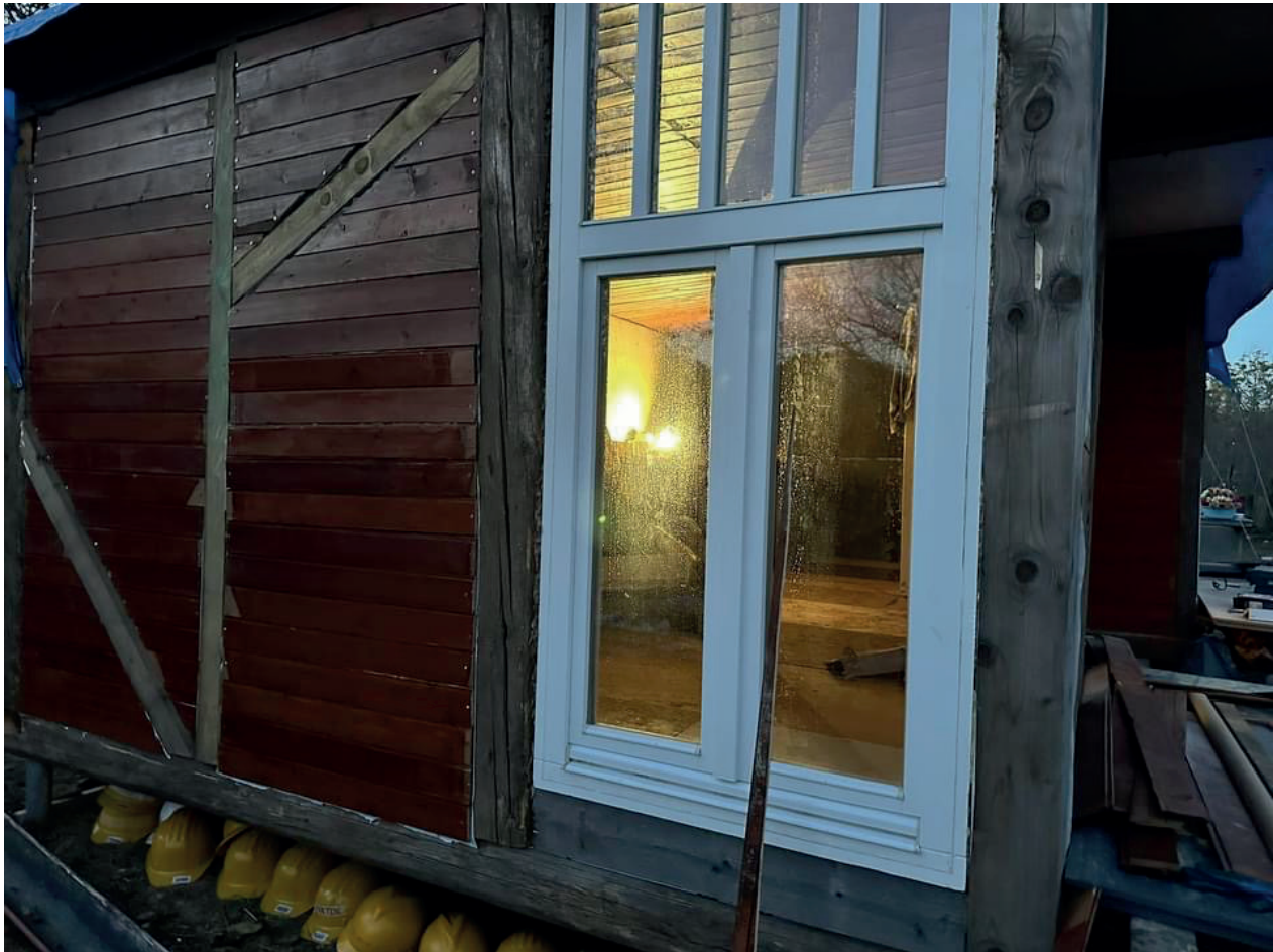
Fig. 4. Fachwerk framework filled with reused wainscoting and heat insulation. The window came from a hotel under refurbishment.
