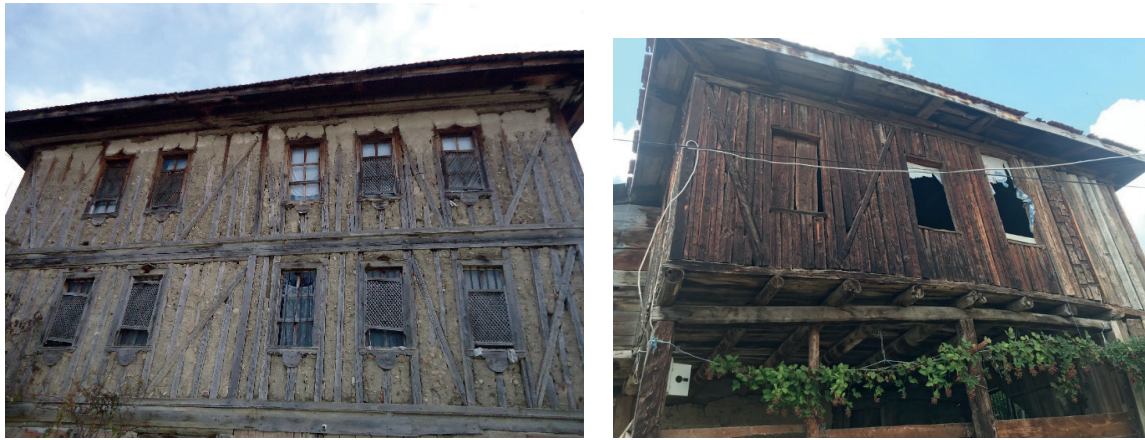
Fig. 4. (a) Adobe filling technique between wooden frame (Medinegil house); (b) timber infill wall between timber frame (Camadan house)
