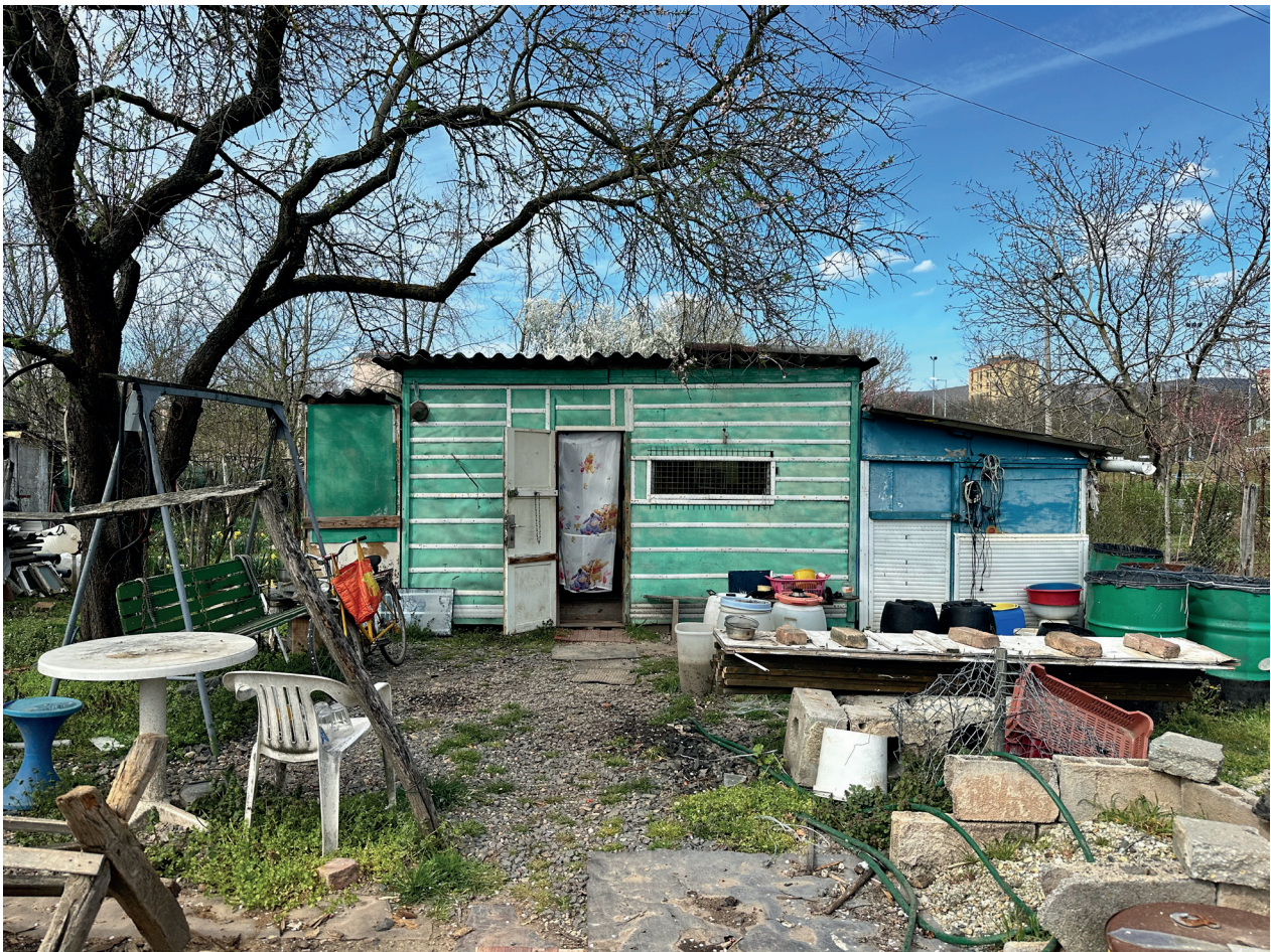
Fig. 2. Self-made house, made of door panels, covered with PVC sheets and plastic shutter
