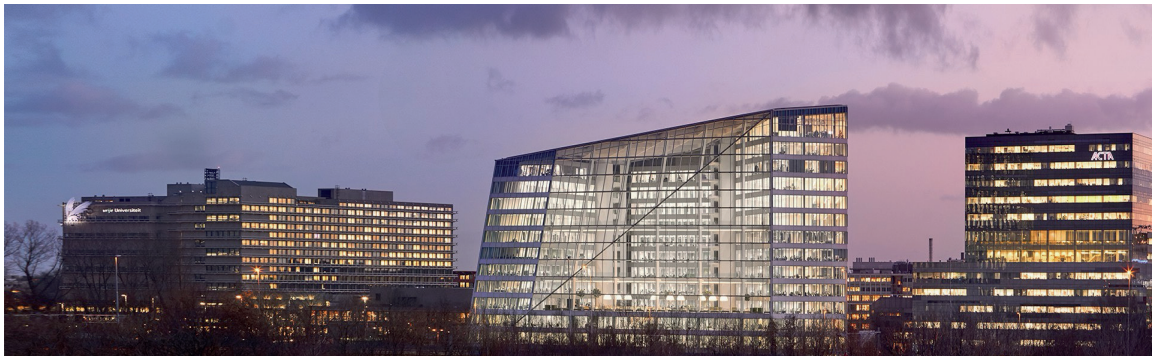
Fig. 3. The Edge (middle), transparent 15 floor atrium [15].
