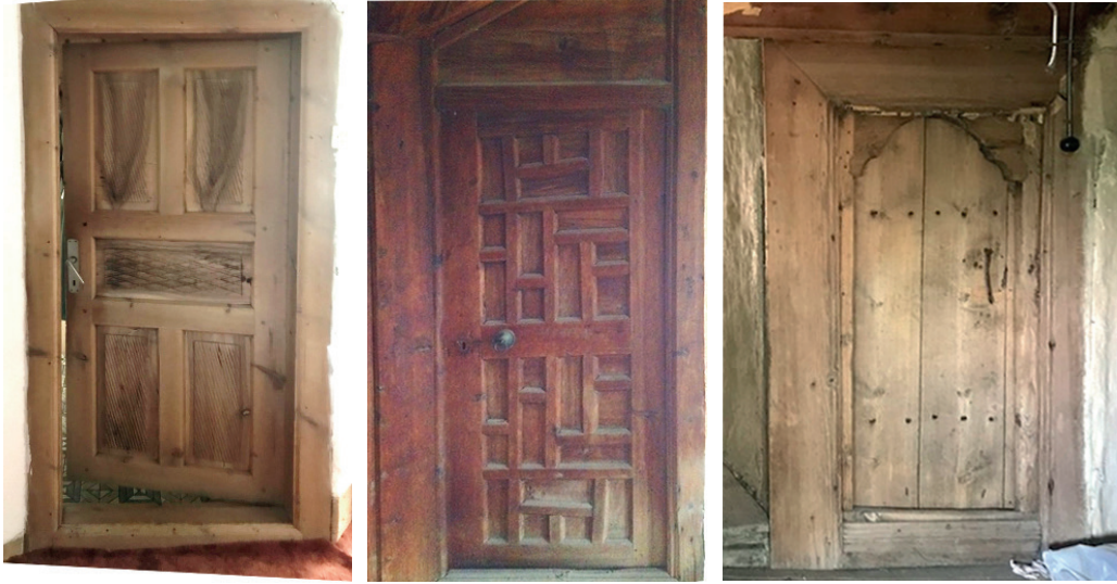
Fig. 12. (a) 5-panel door; (b) the door is decorated with various geometric shapes; (c) the door with a hood
