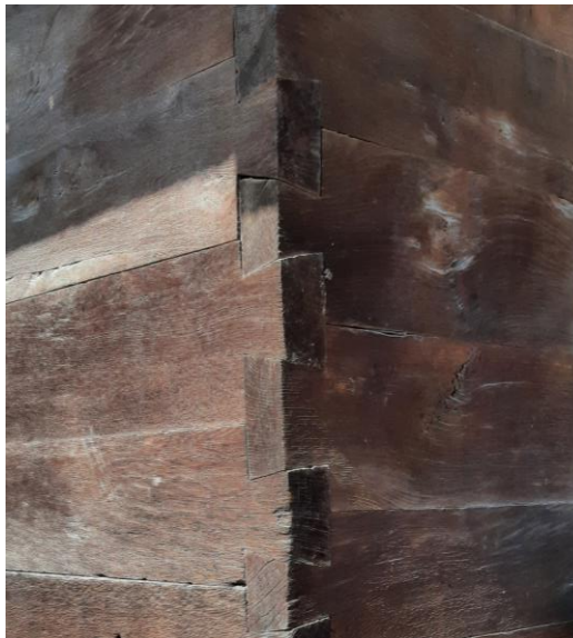
Fig. 4. German angle joint
