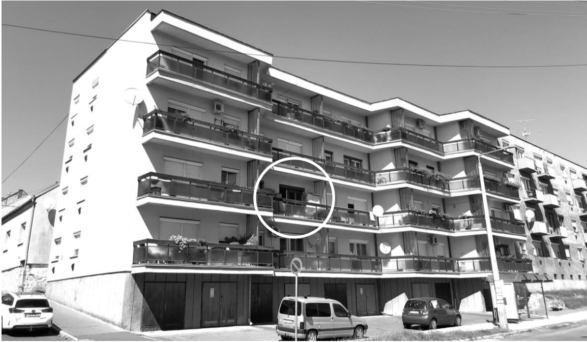
Fig. 1. Well oriented building with shaded windows
