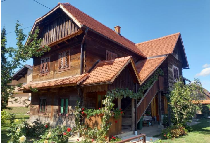
Fig. 5. Traditional timber house in Mraclin: Jerbekov čardak Massive timber walls are constructed with dovetail joints while gable has a lighter structure (Photo by Ratko Cvetnić)
