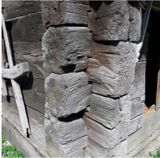
Fig. 3. Croatian angle joint
