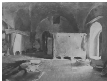
Fig .17: Picture from inside the traditional Palestinian home, showing the mud partition. [14].
