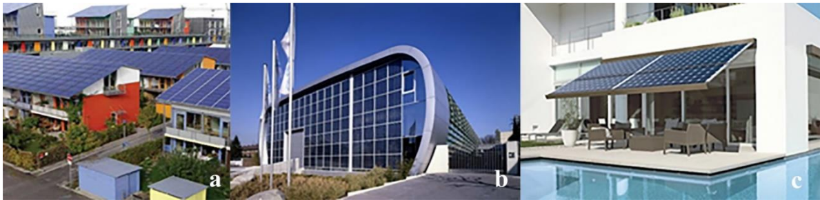
Fig. 1. A different application of BIPV: (a) rooftop; (b) façade cladding; (c) solar shading device. Source: adapted by authors from Google Search Engine.
