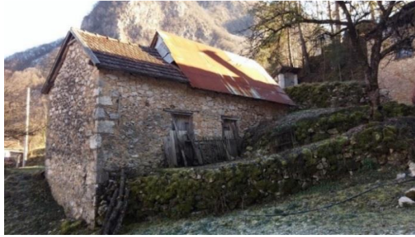
Fig. 4. House contextualization and integration into slope, Ibar.
