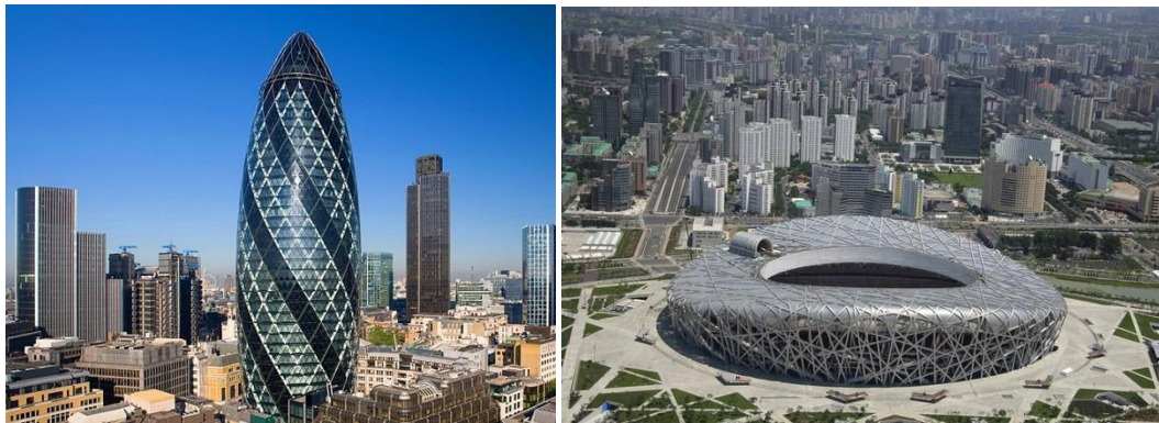
Figure 1. (a) Gherkin building, London, the UK, (b) Beijing National Stadium, Beijing, China.
