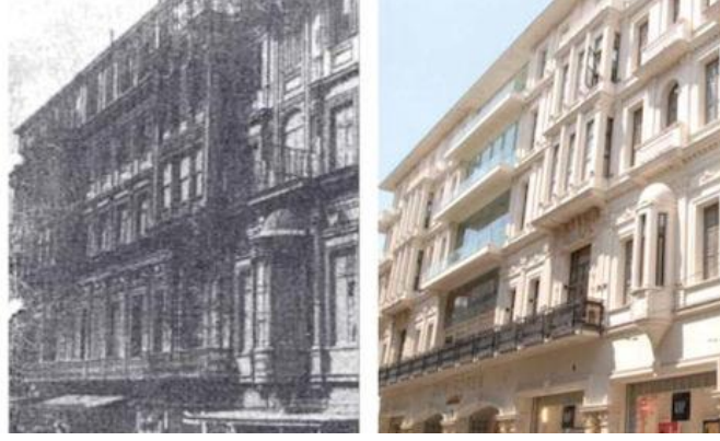
Fig. 3. (a) Deveau Apartment, 1890. (b) Demirören Shopping Mall, 2016.
