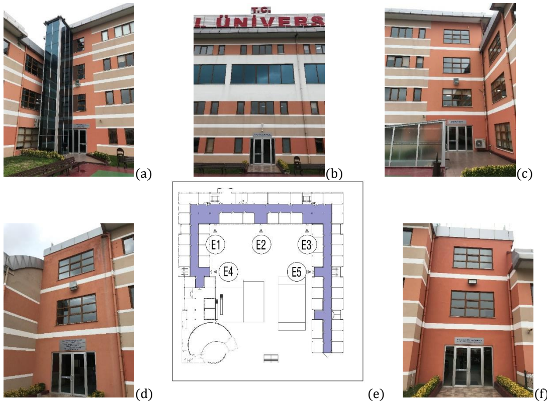
Fig. 3. Entrance Views from Courtyard to the U-shaped the University Building Main Corridor:
