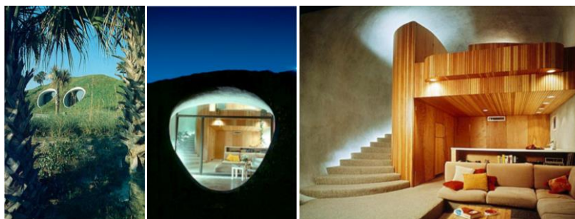
Fig. 1.1.2 (a) External View of the Dune House, William Morgan Architecture, Florida, 1974 [ULR 5]; (b) Outer Appearance of the Dune
