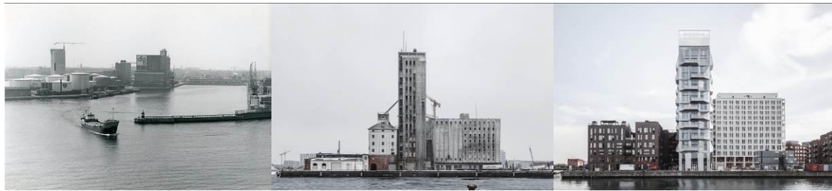
Fig. 1. (a) Old Nordhavn; (b) The Silo, before transformation; (c) The Silo, after transformation
