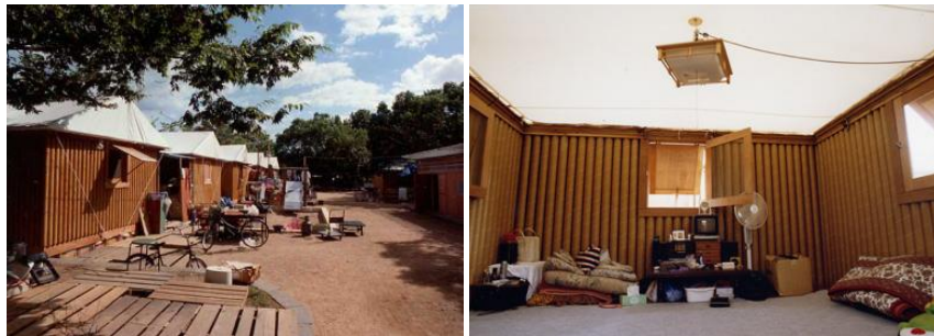
Fig. 1.1.4 (a) Disaster Shelters (Houses), Made of Paper Tubes, Shigeru Ban, Kobe, Japan, 1995 [ULR 8]; (b) Interior Space of Disaster Shelters, Made of Paper Tubes [ULR 8].
