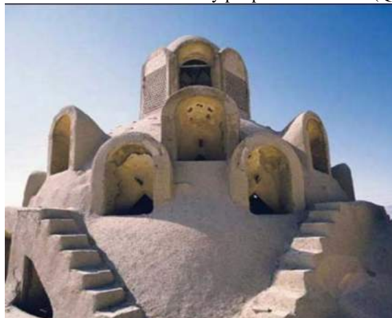
Fig. 5. Badgirs of Boroujerdi house in Kashan
