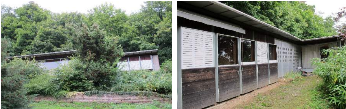
Fig. 1. (a) The Prouvé House in Nancy, France, nestled into the hillside; (b) Facade of the west wing of the house, where the bedrooms are located; the aluminum facade with portholes encloses the bathroom and entrance hall; the living room can be seen in the far-right.
