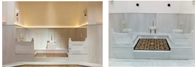
Fig. 8 The iwans and basins of the men's hot space (left) and the iwans and basins of the women's hot space (right) following restoration (photographs: the author's archive)
