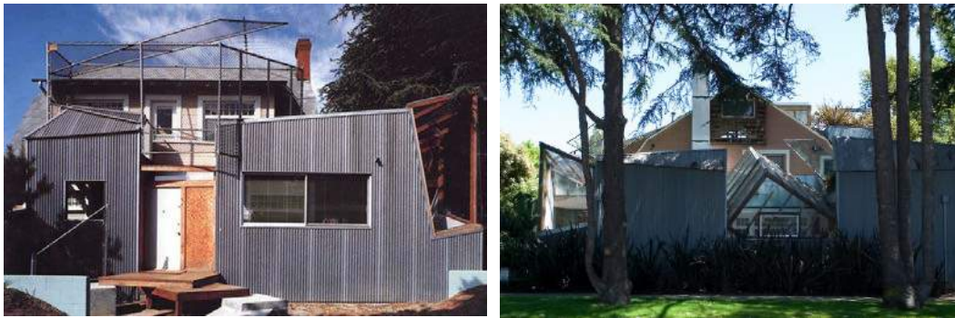
Fig. 5. Gehry House, Frank Gehry, Californiya, 1978 [25].
