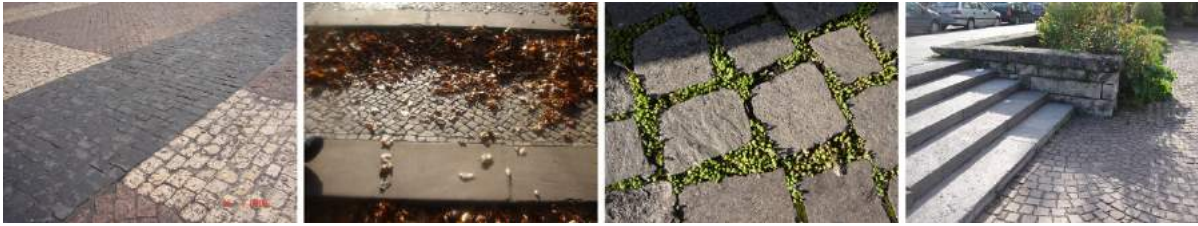
Fig. 3. Permeable flooring examples
