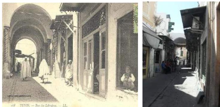
Figure 1: (a) Librarians bazaar (Al-Kotbia Souk) in 1903, (b) Librarians bazaar (Al-Kotbia Souk) presently (a), (b) by author on 15 th of August 2016
