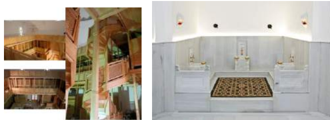
Fig. 13. a- Views from the changing cabins that were renewed during the final restoration made at the Hagia Sophia Haseki Hürrem Sultan Bath b- The sultan iwan at the men's hot space of the bath.
