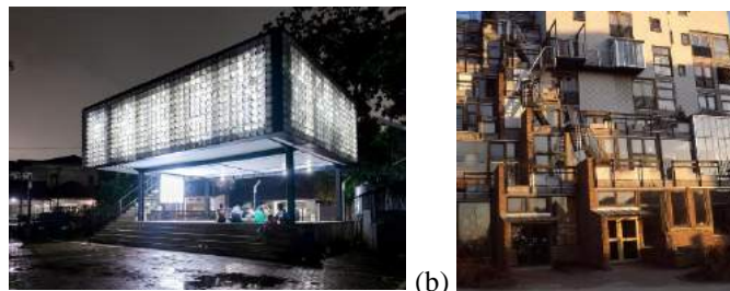
Fig. 8. (a) On the left; Micro Library, Architectural Office: Shau, Kampung-Indonesia, 2012. The facade gives most economical solution to the narrow budgeted project group by consisting 2.000 of ice-cream cups [28]. On the right; Louvain Student Housing facade, Lucian Kroll, Louvain, 1976 [26].
