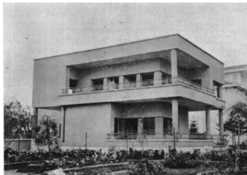
Fig 7. View of House of İhsan Sami
