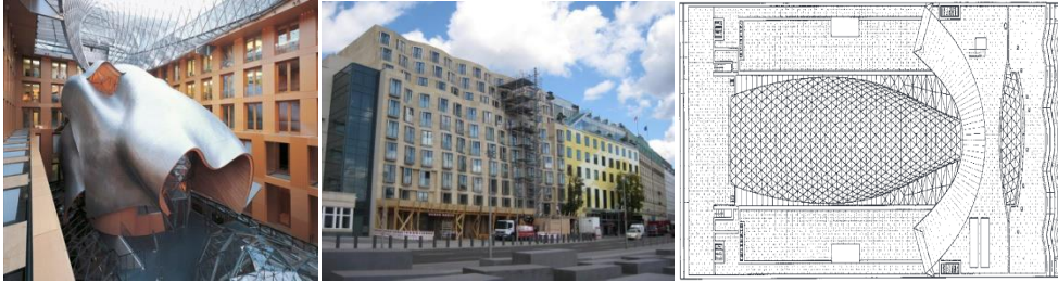
Figure4: The interior space and external pictures of DZ Bank building ( https://www.google.com.tr/webhp?sourceid=chrome-instant&ion1&espv=2&ie=UTF-8=frank+gerhy+dz+bank )
