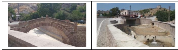
Fig. 8. (a) Stone Bridge; (b) Sille Entrance Bridge
