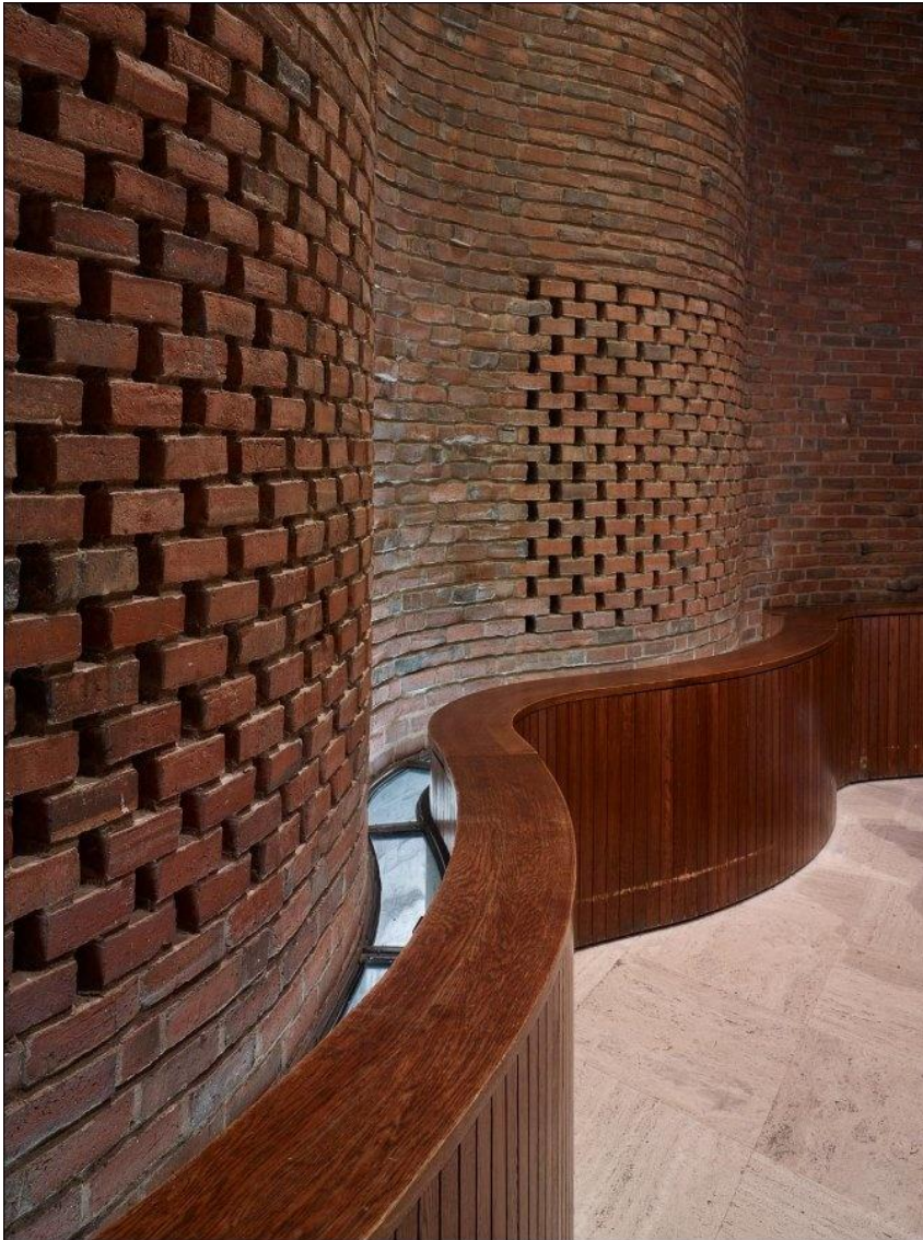
Figure1: Aero Saarinen, Chapel wall. Bricks used as ventilation elements
