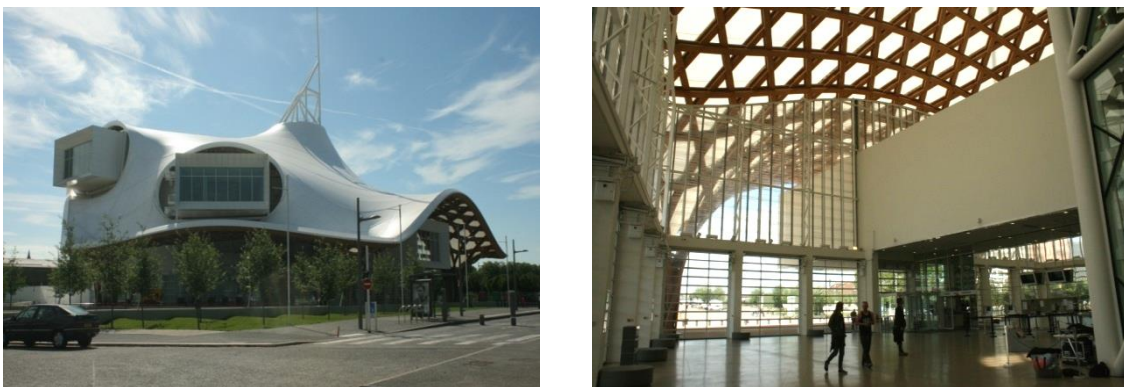
Fig.6. (a) Outer view of Centre Pompidou-Metz; (b) Entrance of the Museum
